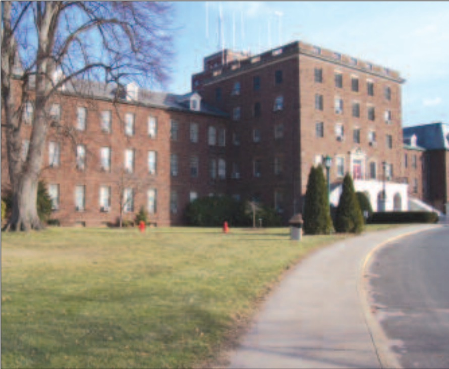
Left, Connecticut Valley Hospital is a sprawling campus. A change in mission led to a change in security strategy. Right Access controls first started as a limited number of doors as the facility started its transformation from keys to cards.
