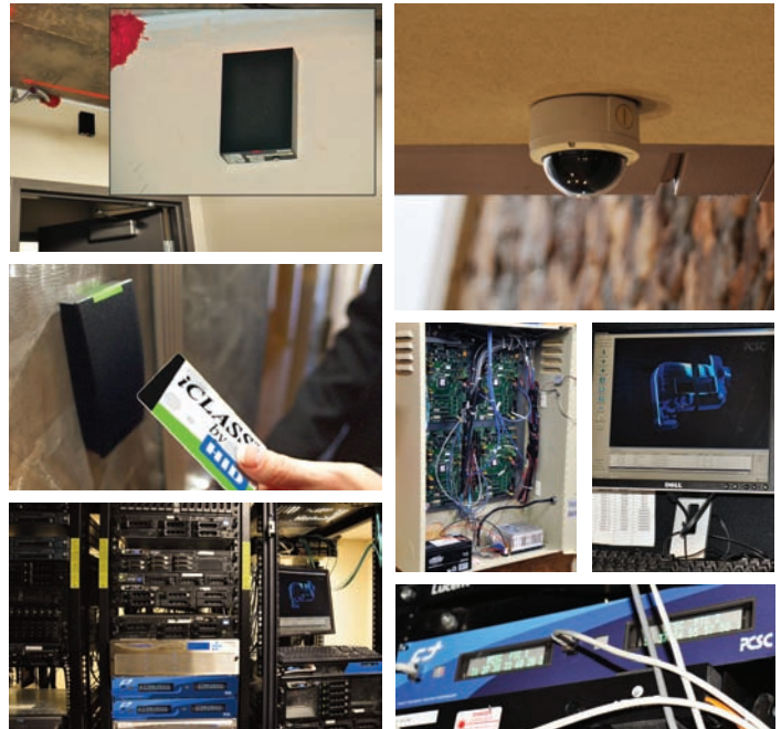
Initial setup and testing of equipment
